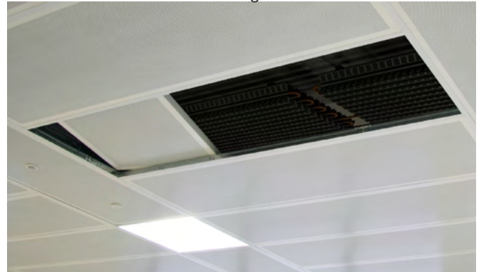
“Hybrid” Radiant / Convective Chilled Beam Ceiling
